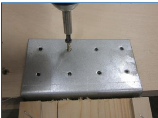
Fig. 41: Fastening the transport ramps
