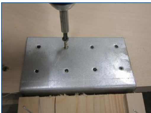
Fig. 17: Fastening the transport ramps
